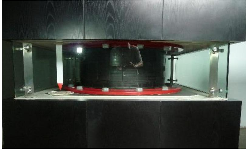
*Figure 4. A circular rubber bearing containing many thin steel plates is located between the bottom of every column and its foundation to isolate the building from horizontal earthquake shaking.*
